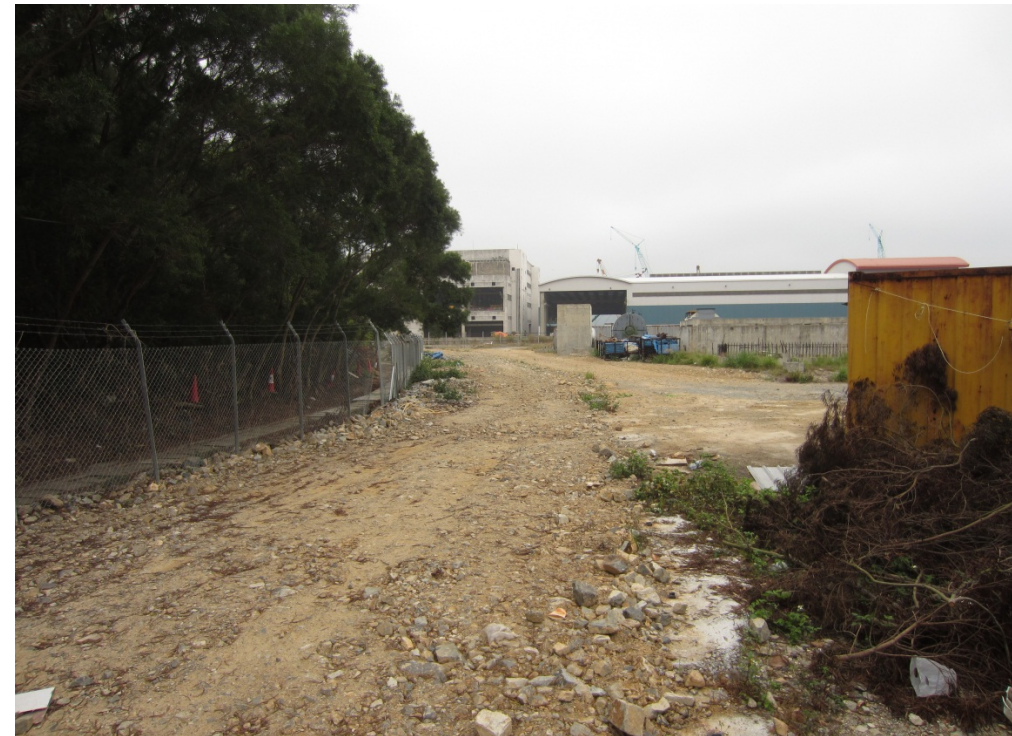
Photo 2 – Hoarding fences of the land duct have been dismantled and the site has been reinstated to its original conditions.
