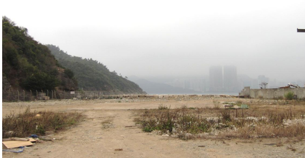
Photo 1 – Hoarding fences of the new beach manhole have been dismantled and the site has been reinstated to its original conditions.
